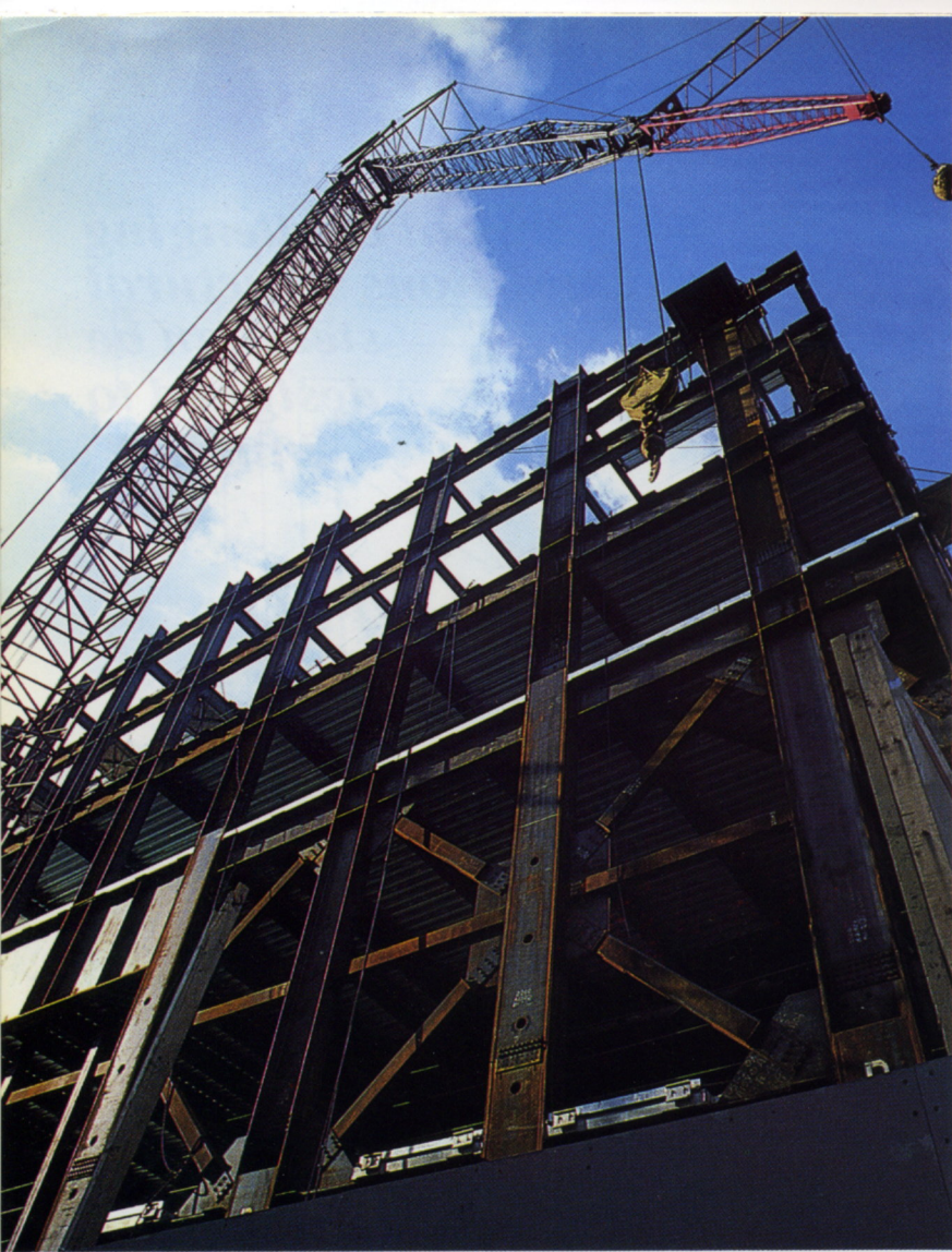
Crawler tower cranes erected steel up to the ninth floor
