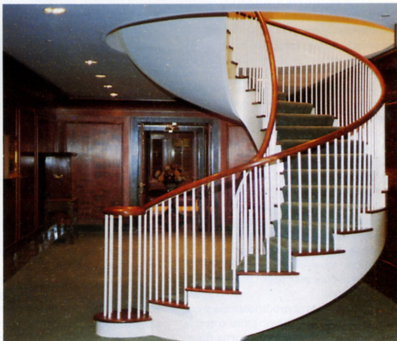
These photos, supplied by Empire City Iron Works, Inc., show the egg-shaped stair as it was fabricated in the firm's Long Island City plant. Below is the finished product. All of the stair's splice plates were welded up and ground smooth before the final wood finish was added.
