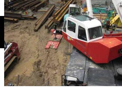
Figure 5: The primary construction crane before the erection of the structural frame. Here, it is positioned in the southeast corner of the site.
