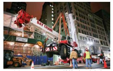
Figure 4: The primary construction crane was lifted from the street level and into the excavated site during the Department of Transportation's sanctioned off-hours.
