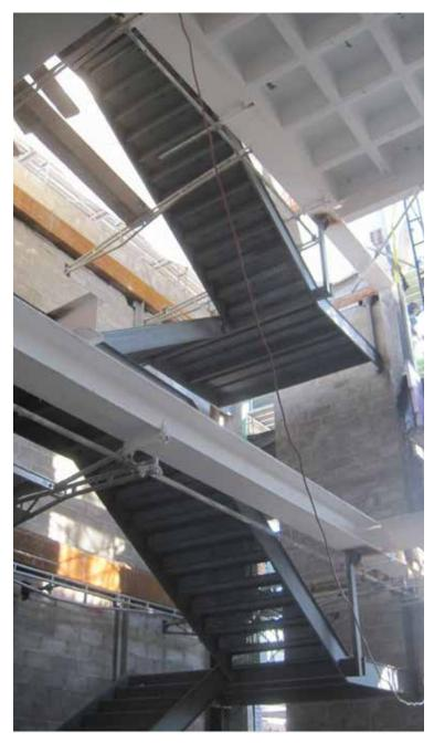
View of the new architectural stair from the ground floor. Underside of the concrete waffle slab is visible on the right.
