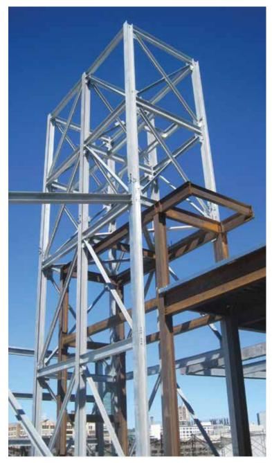
Steel beacon tower with stair bulkhead and superbrace.
