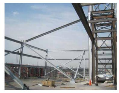
Superbrace framing system for the steel beacon tower.
